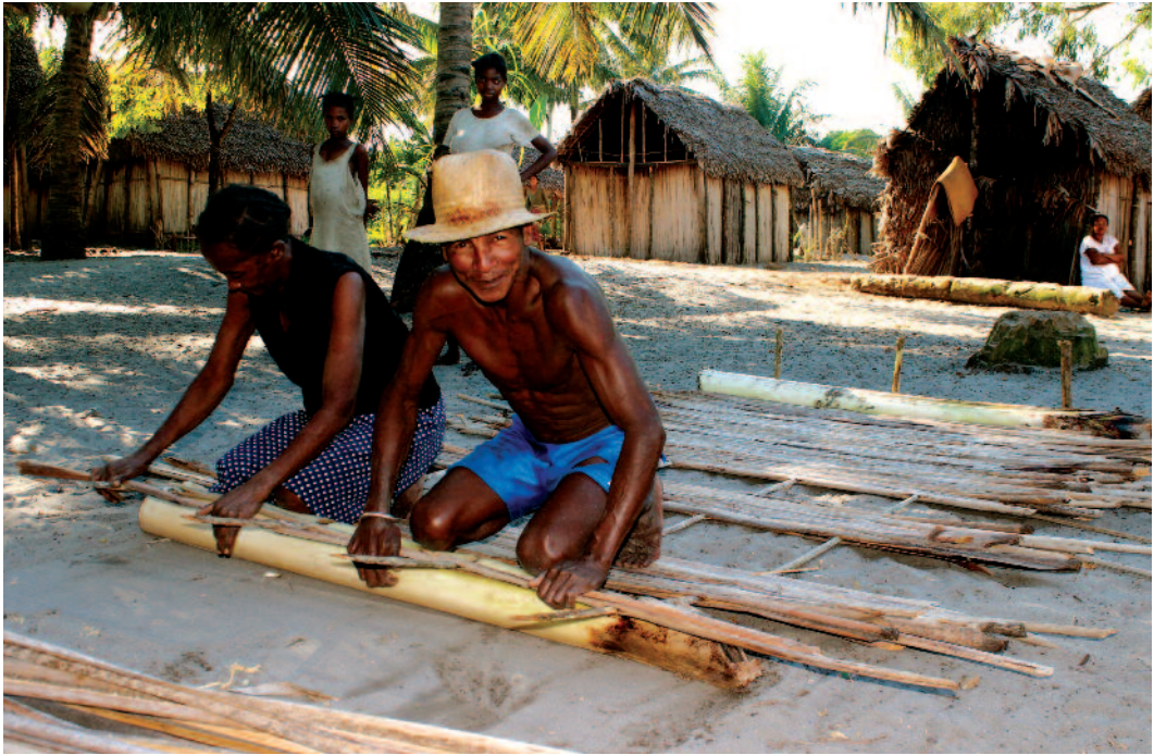
6. Dypsis scottiana stems being used to make wall panels (Photograph by Naidi McDonnell).
