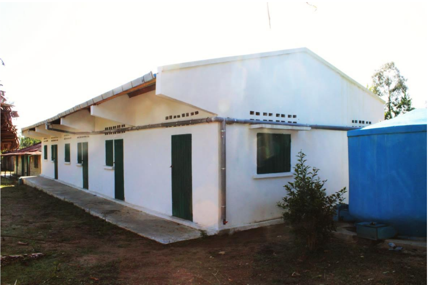
The completed school building and teacher accommodation at Emagnevy Primary School.
