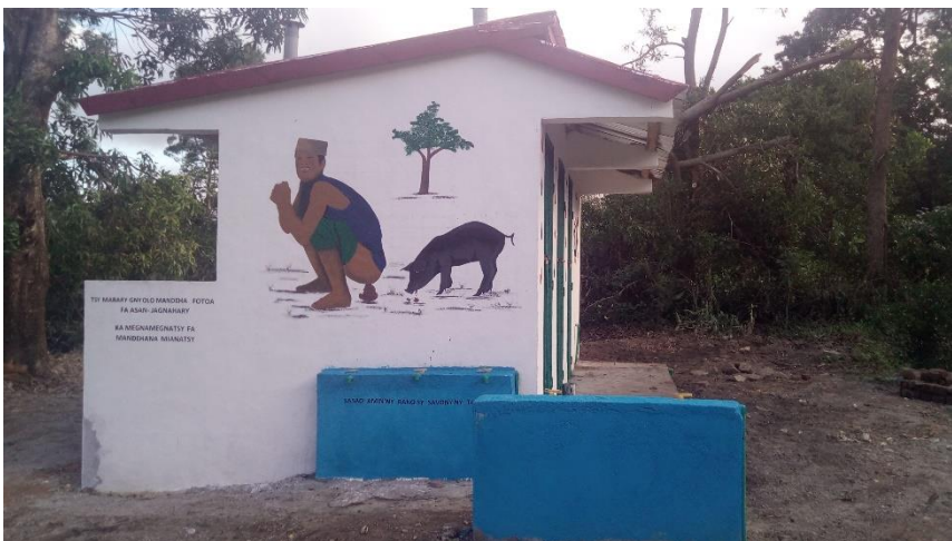
Front view of the newly constructed latrine blocks at Emagnevy Primary School with behavioural nudges (top), side view of the latrine block with mural and handwashing stations (bottom).
