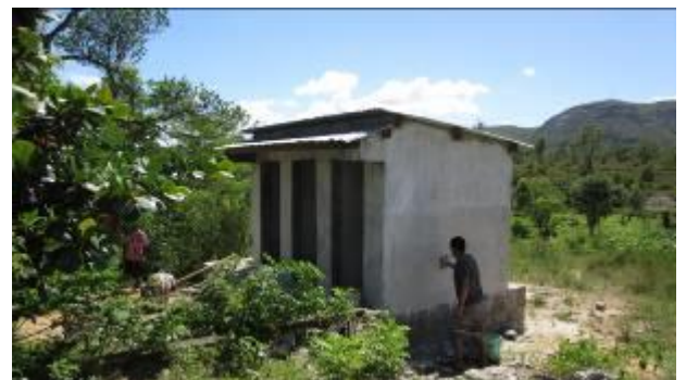
Painting the latrine
