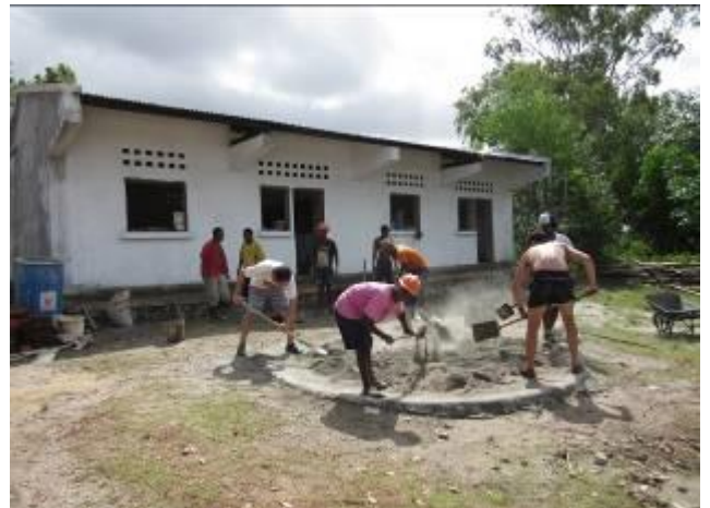
Mixing the final batches of cement outside the new building
