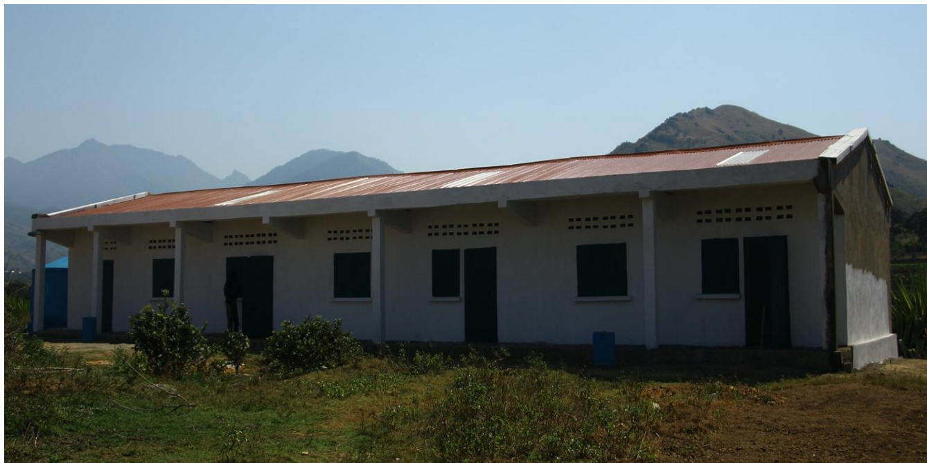
The completed three-classroom school building in Mandiso, with two additional teacher accommodation rooms, and an updated cyclone-resistant design.
