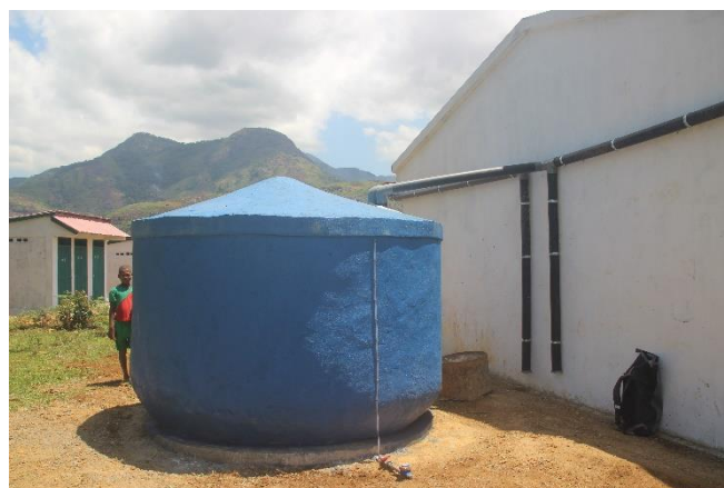
New latrines and handwashing facilities (left) and rainwater harvesting system (right)
