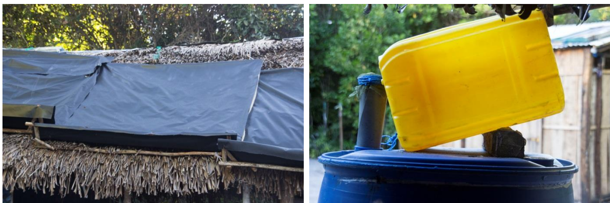
Figure 2: Left: Simple modular roofing allows for easy installation and expansion to improve performance if desired. Right: Overflow first flush system made of a jerrycan maintains high water quality.
