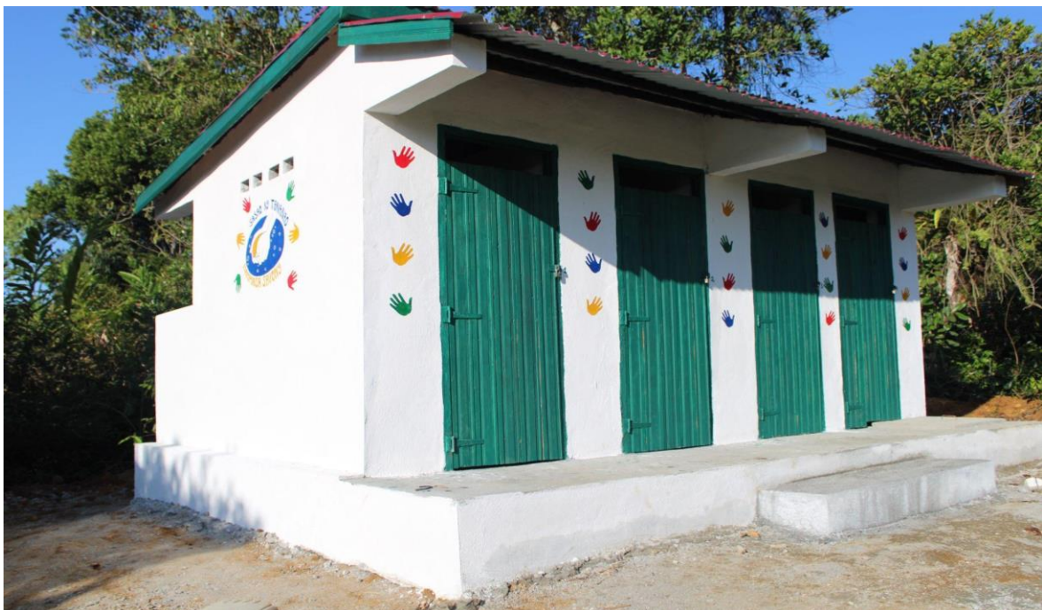
The new latrine block with four gender-segregated latrines.
