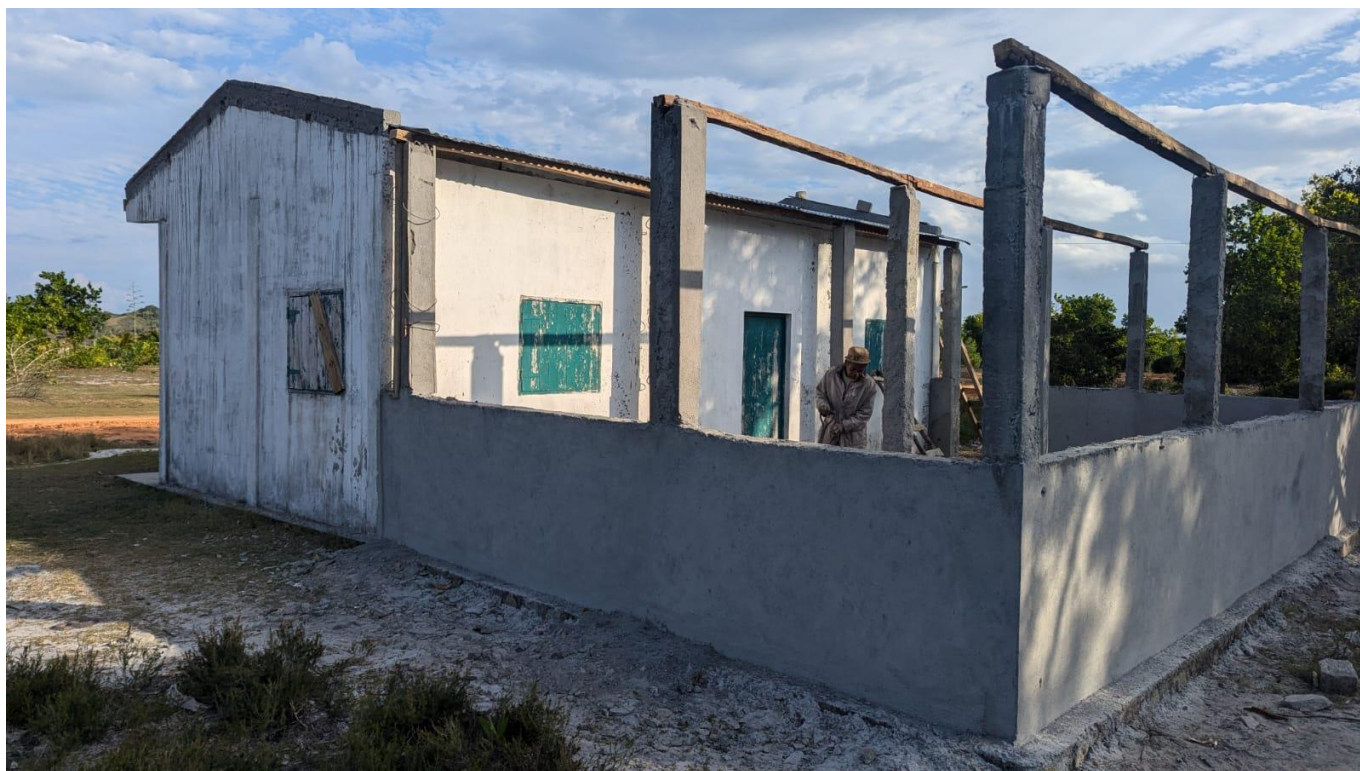
Repairs to the Weavers Workshop in progress, with concrete pillars being installed in the outdoor weaving area to provide further support and stability to the roof.
