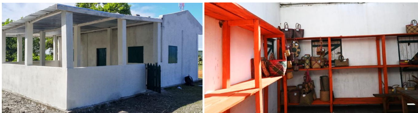
The Workshop's outdoor weaving area fully constructed and repaired, including reinforced concrete pillars (left). The Workshop repaired and ready to showcase new mahampy products (right).
