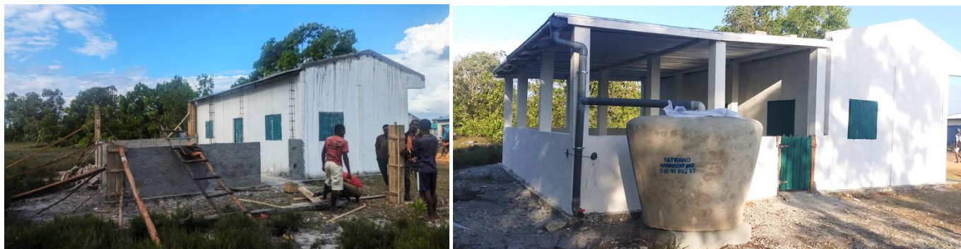
Construction and repair activities ongoing at the Mahampy workshop building (left) and the building complete with a rainwater harvesting system (right).
