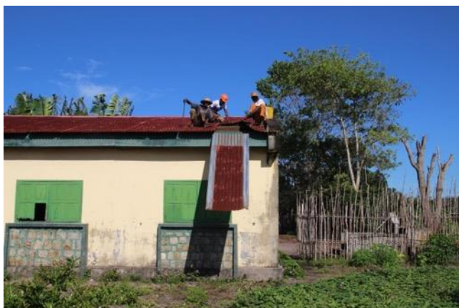
Left: The first sheet of old corrugated metal roofing is removed. Right: The clear contrast between old (left) and new (right) roofing is visible.
