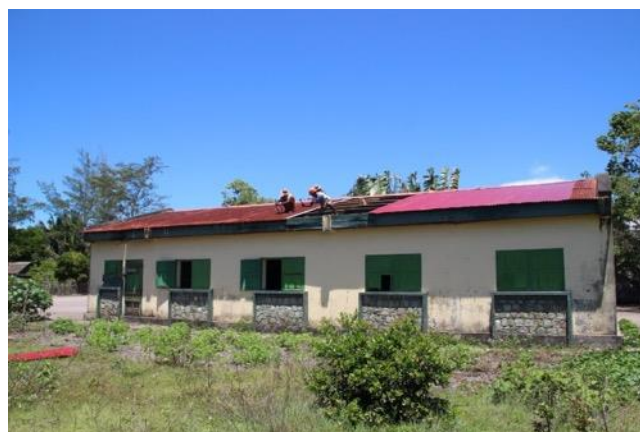
Left: The first sheet of old corrugated metal roofing is removed. Right: The clear contrast between old (left) and new (right) roofing is visible.
