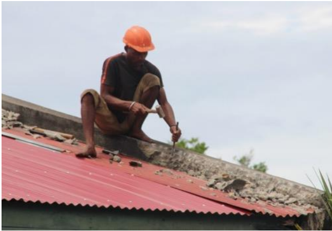
Left: The concrete ends of the roof are chiselled away in order to remove the end corrugated sheeting. Middle: Skilled construction workers fill-in the wooden mould with a concrete mix and new reinforcement. Right: The finished concrete end with the new roofing panel in place.
