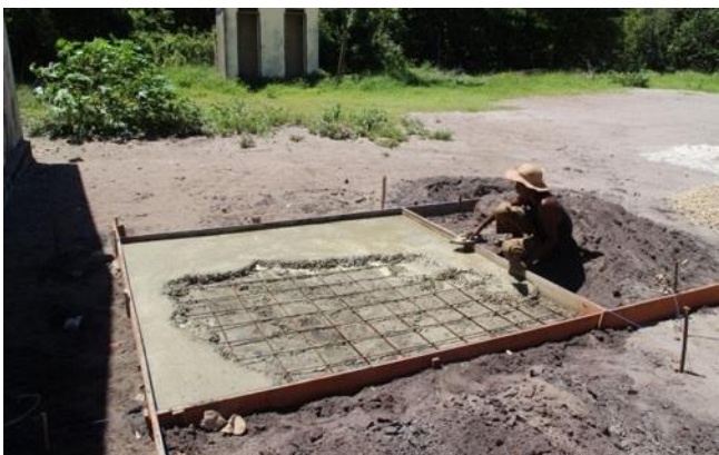
The stages of construction for the first tank foundation.
