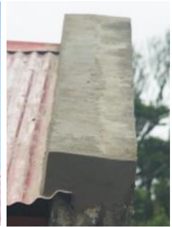
Left: The concrete ends of the roof are chiselled away in order to remove the end corrugated sheeting. Middle: Skilled construction workers fill-in the wooden mould with a concrete mix and new reinforcement. Right: The finished concrete end with the new roofing panel in place.
