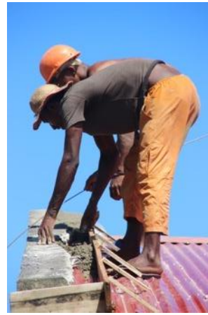
Left: The concrete ends of the roof are chiselled away in order to remove the end corrugated sheeting. Middle: Skilled construction workers fill-in the wooden mould with a concrete mix and new reinforcement. Right: The finished concrete end with the new roofing panel in place.
