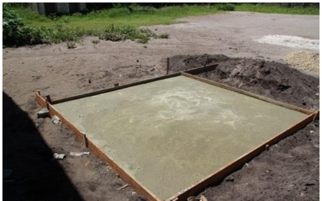
The stages of construction for the first tank foundation.
