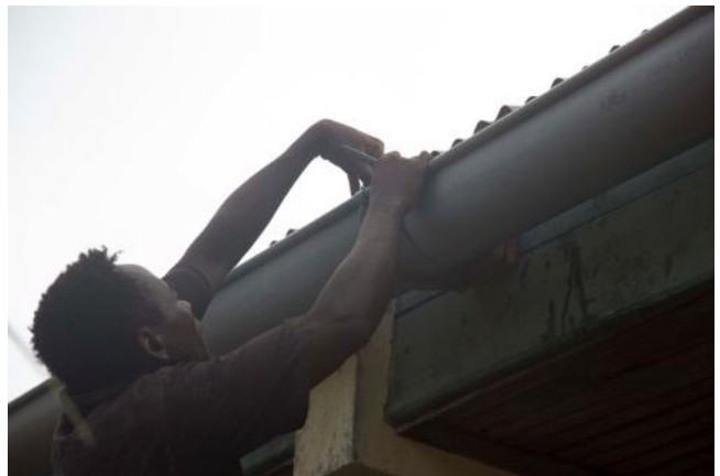
Left: One of the 16 gutter brackets needing adjustment for perfect water flow to the tanks.
