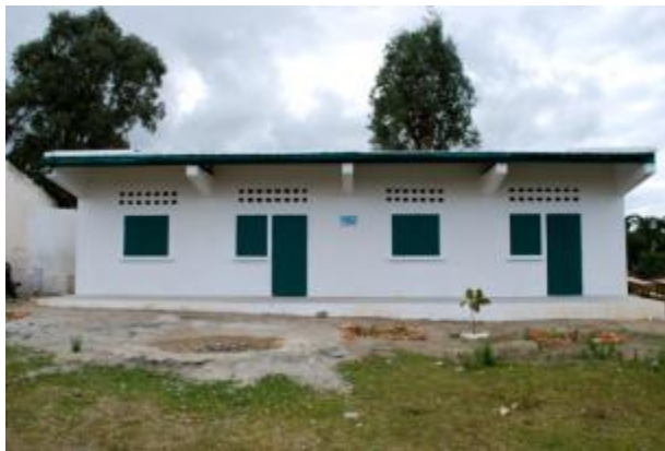
The completed school building and rainwater harvesting tank (on the left)
