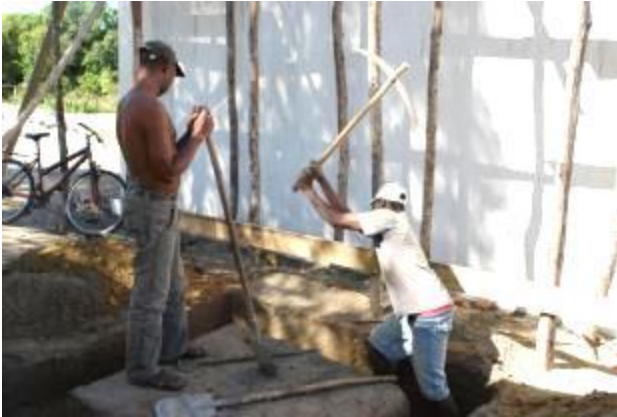
Foundations are dug for the rainwater harvesting tank
