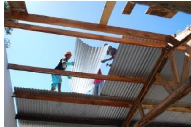
Corrugated iron roof laid by the construction team
