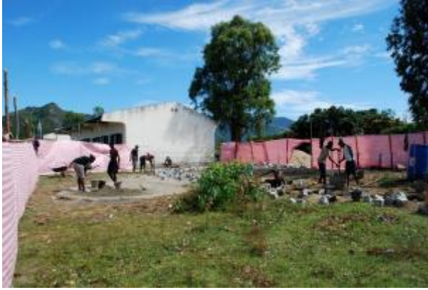
Site fenced off, marked out and ground cleared
