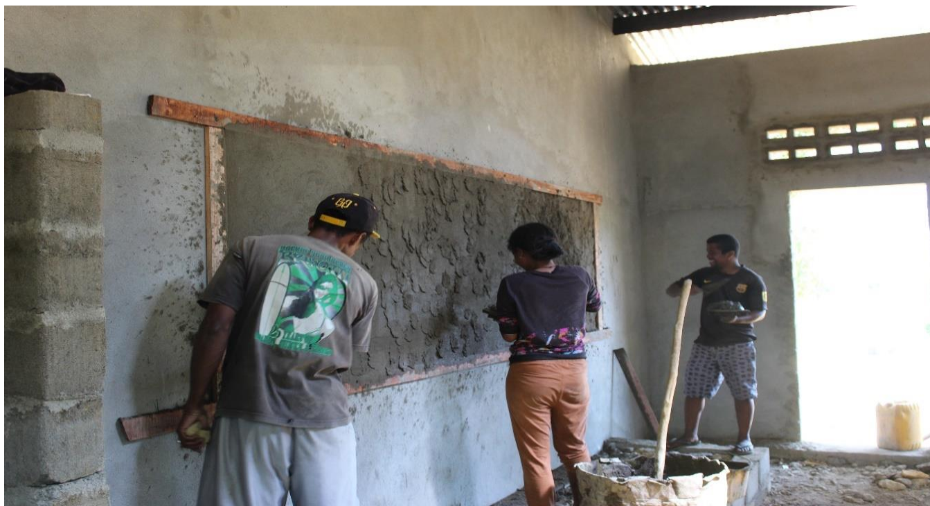
Construction of the blackboard.
