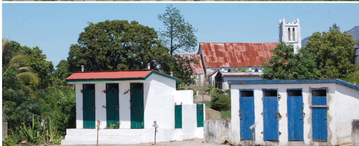
The newly-constructed WASH infrastructure next to Lanirano (above) and Manambaro (below) Primary Schools' existing facilities
