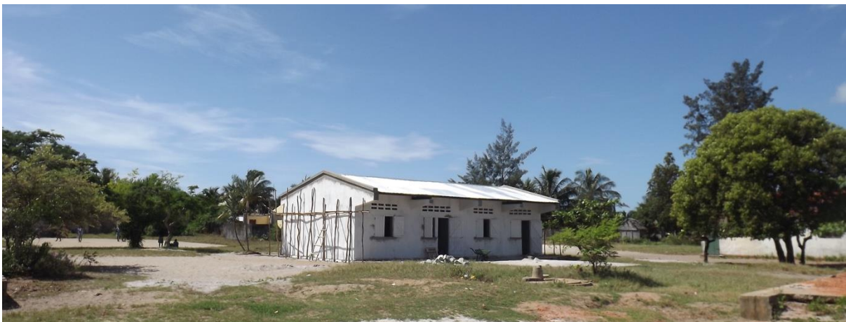
The new classroom building in Lanirano Primary School in early January 2019
