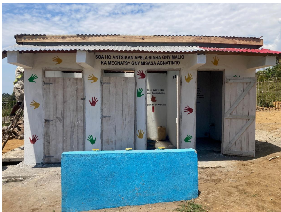
Newly built latrine block with accompanying handwashing station.
