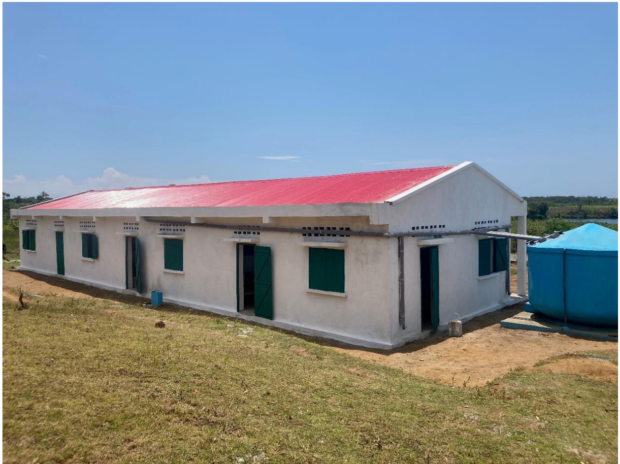
View from the back of the school building, along with the 10,000 litre rainwater harvesting system.
