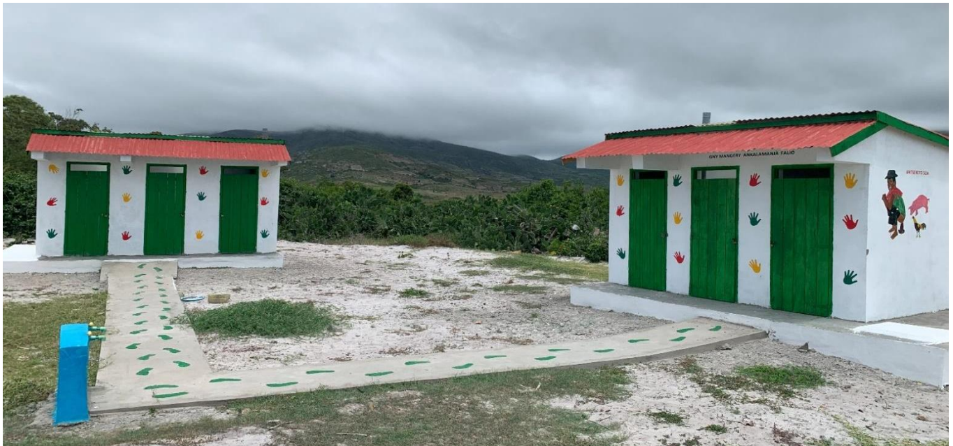
Gender-segregated VIP latrines with an MHM facility and handwashing station at the lower secondary school.
