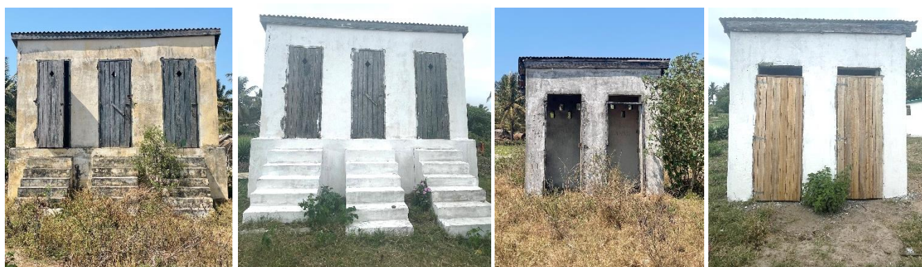
Before and after of the repaired latrines at Sarisambo Primary School.
