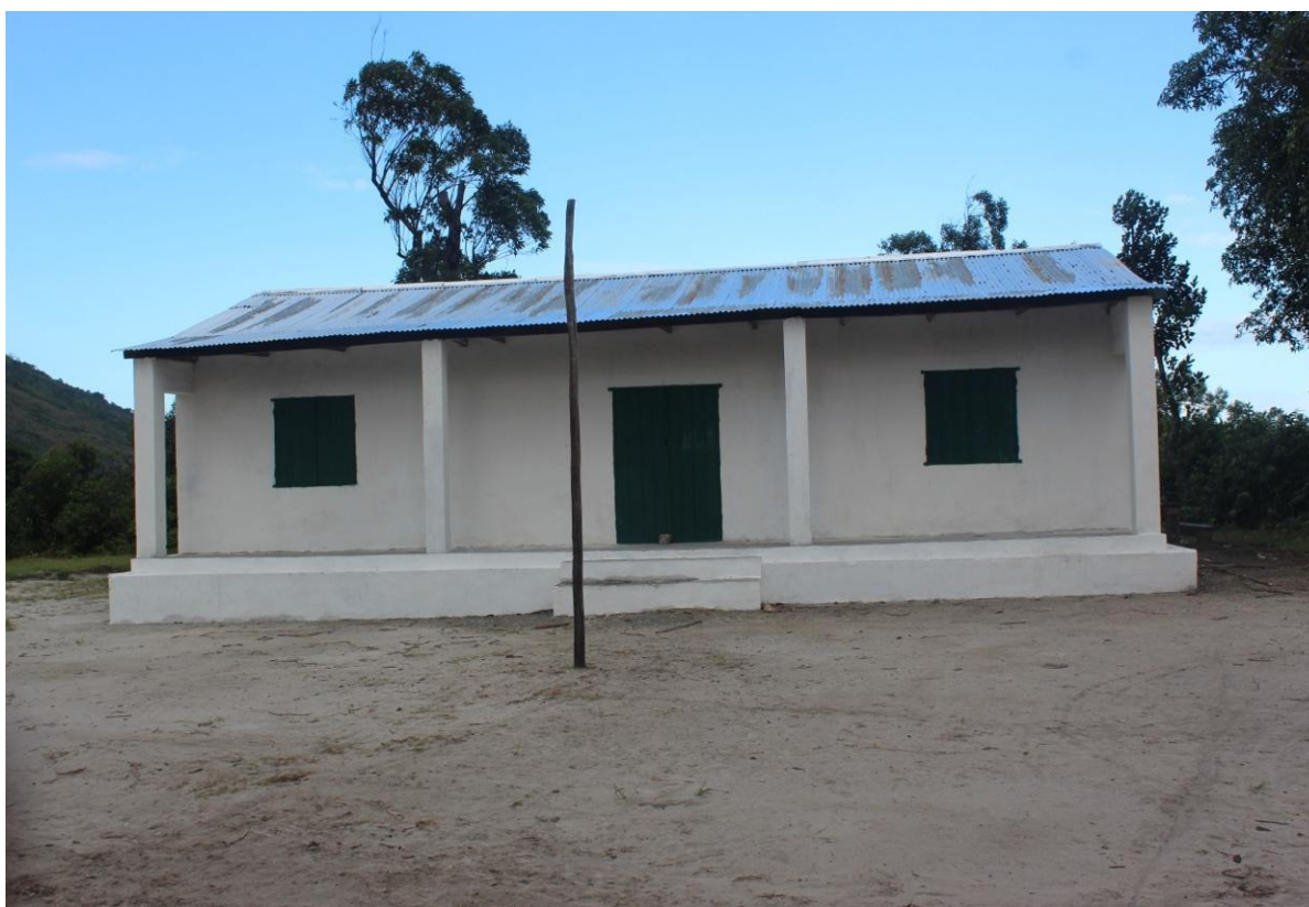
Repaired classroom at Vatambe Primary School
