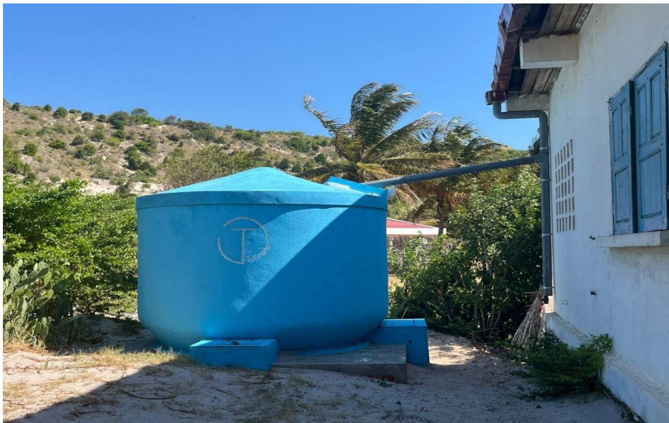
The 10,000-litre rainwater harvesting system installed at Ambinanibe CSB.
