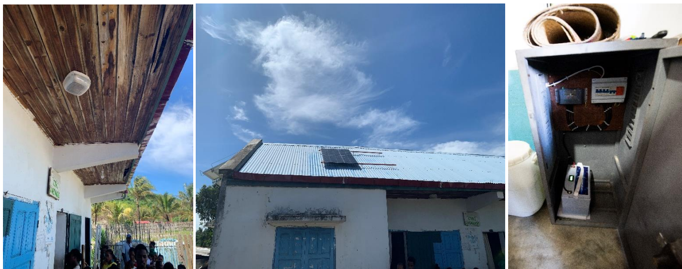
The fixed lumen bulbs above the veranda of the CSB (left), the solar panels installed on the CSB roof (center), the solar generator inside of the access panel (right).
