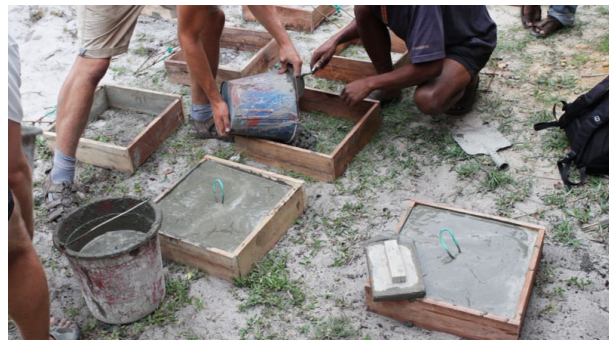
Azafady's Pioneer volunteers pour concrete to produce anchors for buoys
